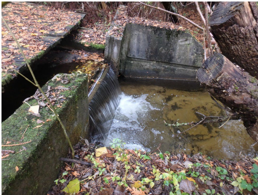
Photo 10: Photo showing the old dam located in Habitat Zone 1 near the inlet to the pond showing the dam and plunge pool. (Photo Date: October 22, 2020)
