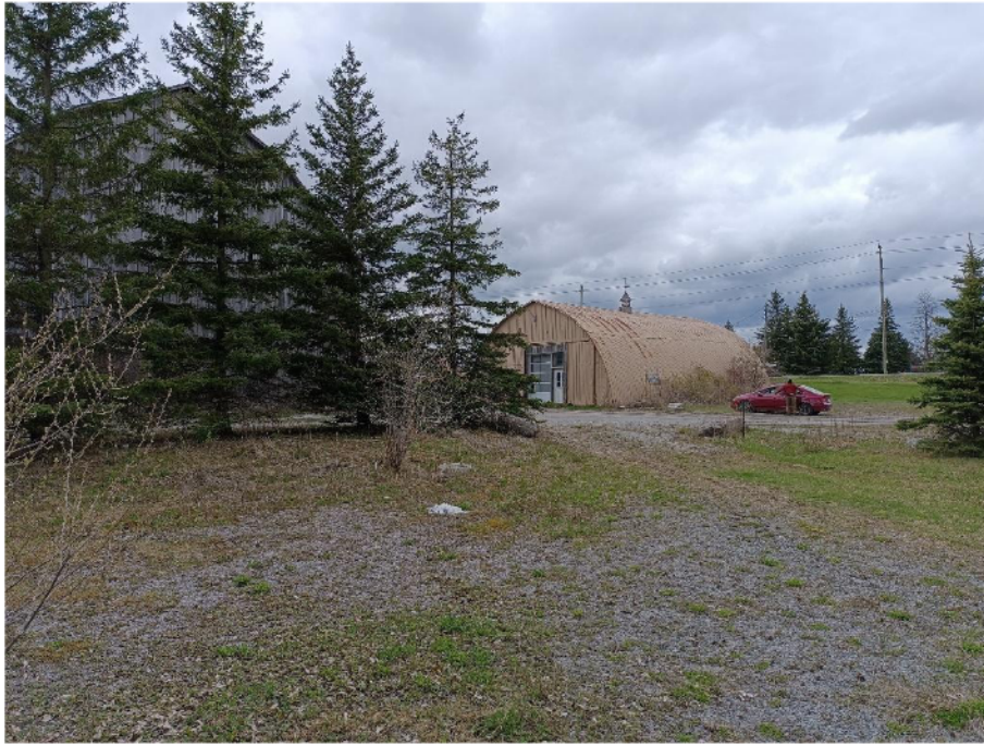
Image 5: Disturbed areas around modern structures.
