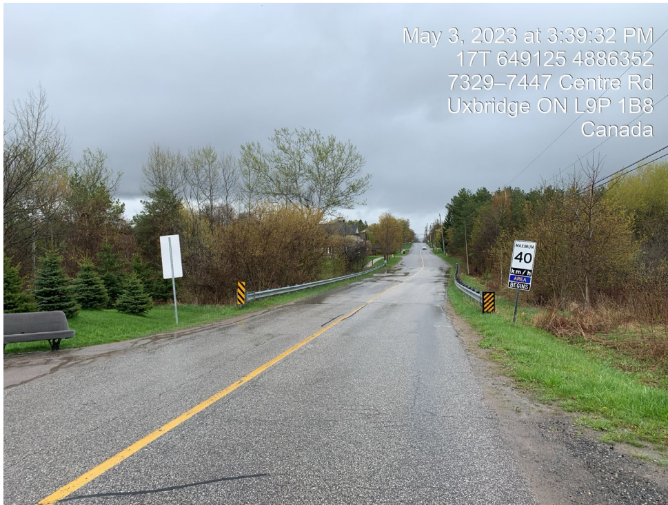
Photo 7 - View along Centre Road to the south.
