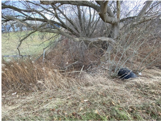
Photograph 9: DF1 - Ephemeral feature north of property, looking east from Centre Road.
