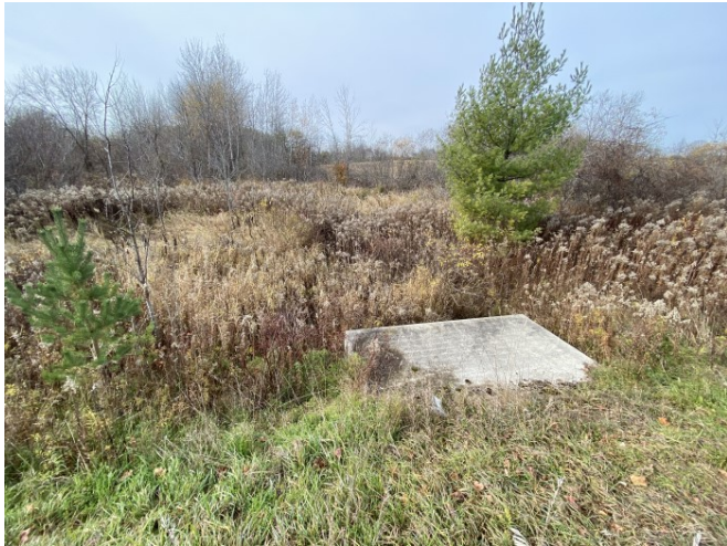
Photograph 1: Uxbridge Brook Tributary, looking upstream on west side of Centre Road.
