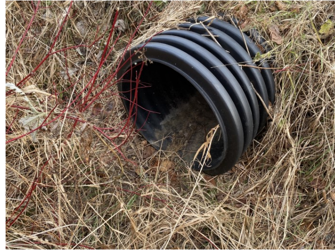
Photograph 12: DF1 - Ephemeral feature north of property, culvert inlet at Centre Road.
