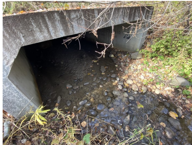
Photograph 2: Uxbridge Brook Tributary, looking upstream at Centre Road culvert outlet.
