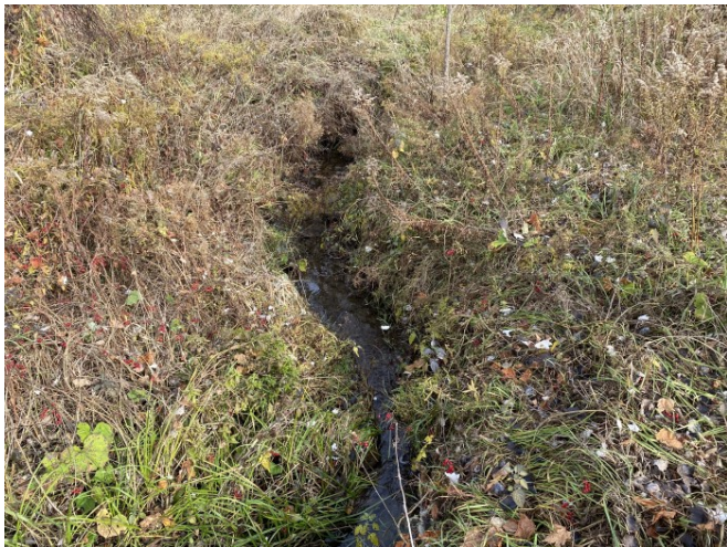
Photograph 3: Uxbridge Brook Tributary, looking downstream near Centre Road culvert.
