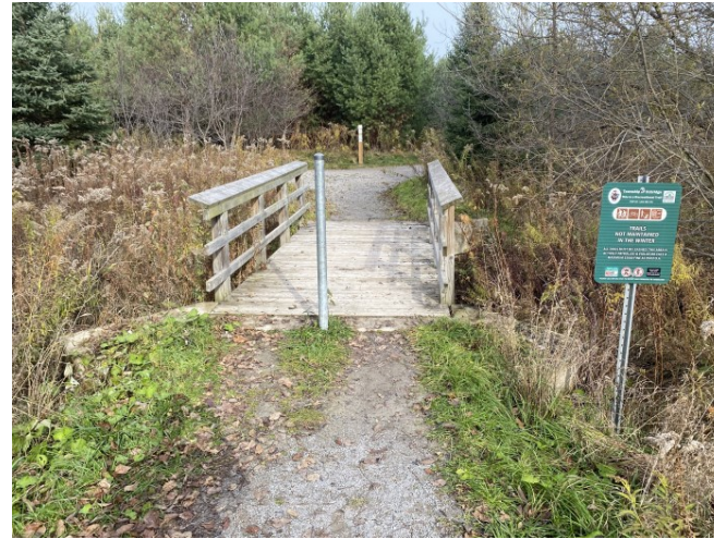
Photograph 6: Uxbridge Brook Tributary, typical foot bridge structure.
