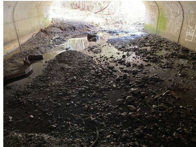
Photograph 8: Uxbridge Brook Tributary, looking downstream inside arch culvert at Oakside Drive.
